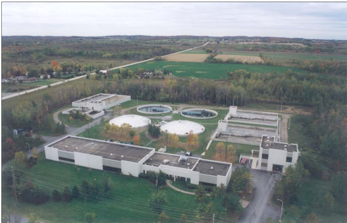
Figure 18-1 Existing Lakeshore WPCP Photo
